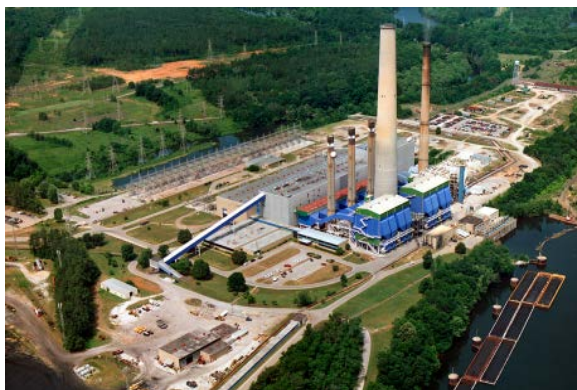
TVA Colbert Power Plant Huntsville, AL - DEC 1998
